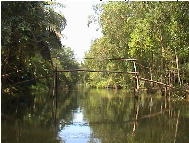
Image 18: Bamboo bridge in the Southwest region of Vietnam Source: Author
